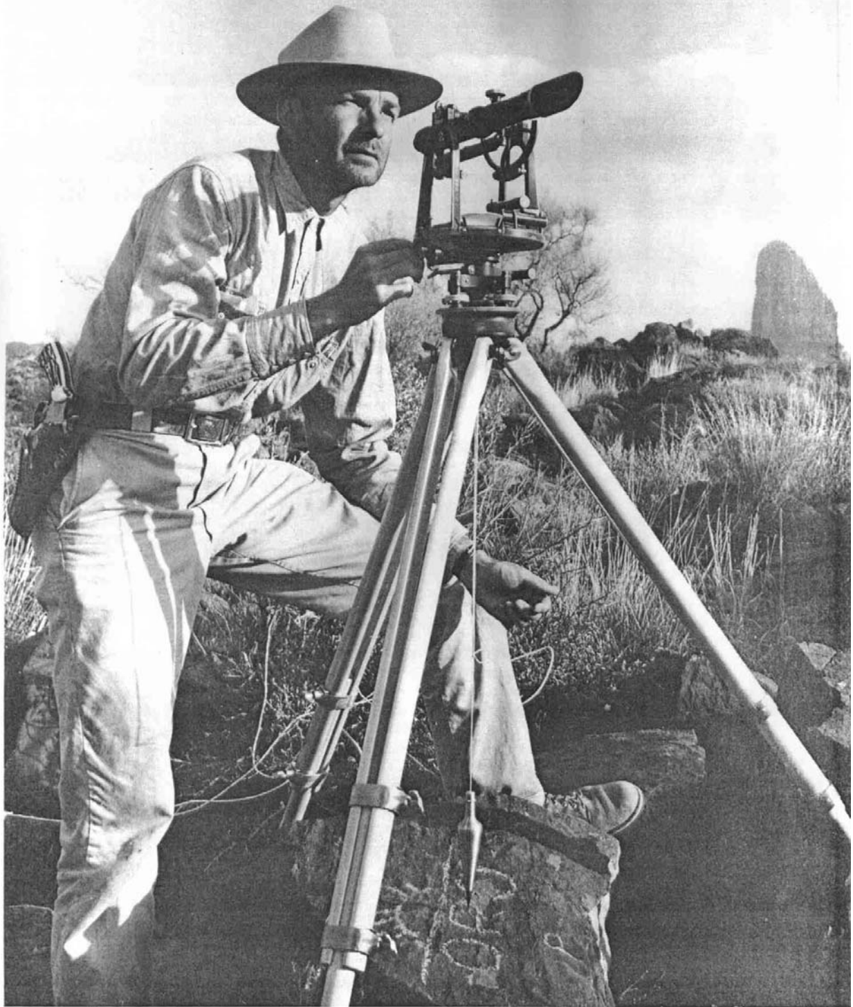
The author reworking the Salazar survey, April, 1949. Note the Miner's symbols on the rock directly beneath the instrument. This spot marked the northwest end of the presumed triangulation base leg atop Black Top Mountain. Nyle Leatham photo.
